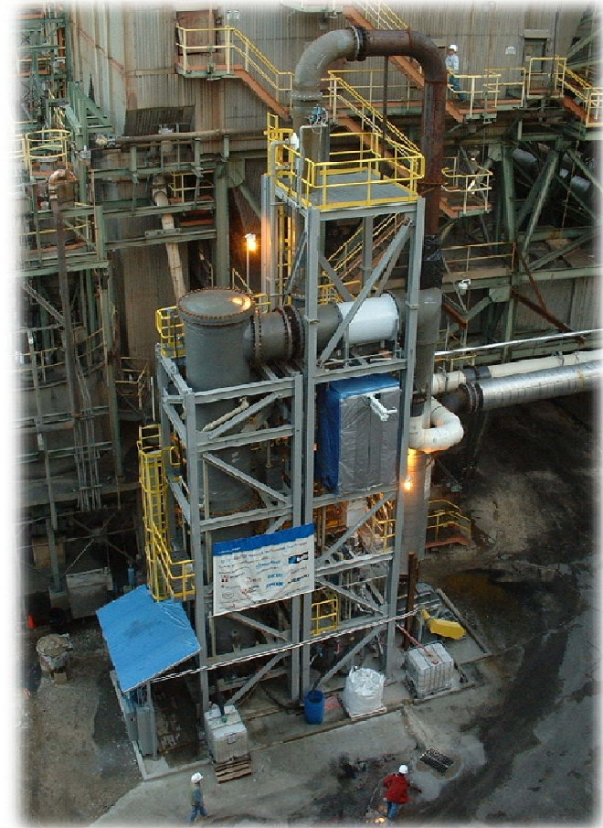
Mercury Research Center Pilot wet FGD
